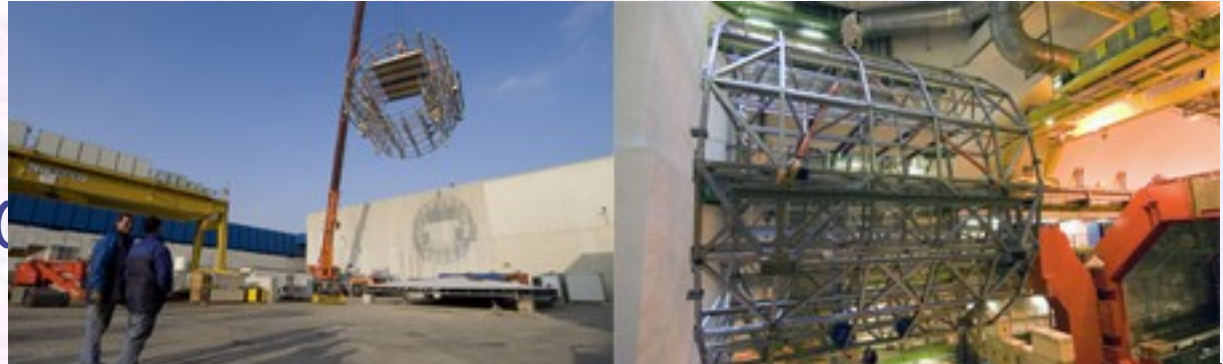
In February 2006 Alice Space Frame was lowered into the pit
