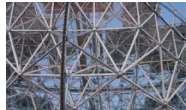
Examples of the space-frame construction. H.E.S.S. steel space-frame (up) and the MAGIC three-layers CFRP space-frame (down).
